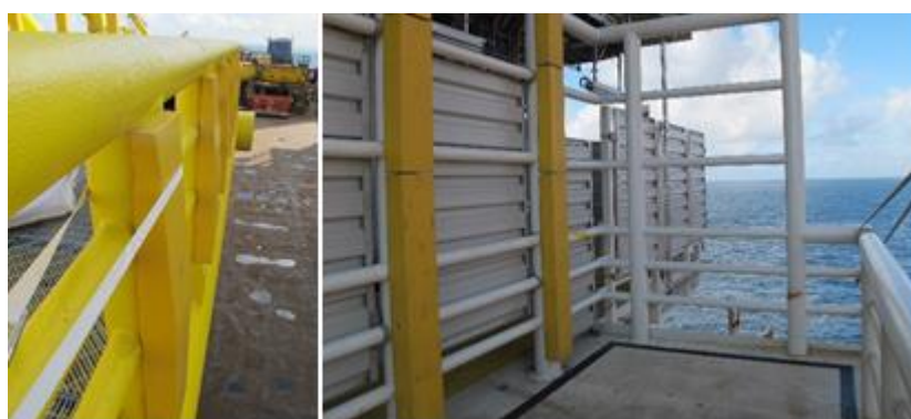
Figure 6.6 Example of bumper and guide structures
