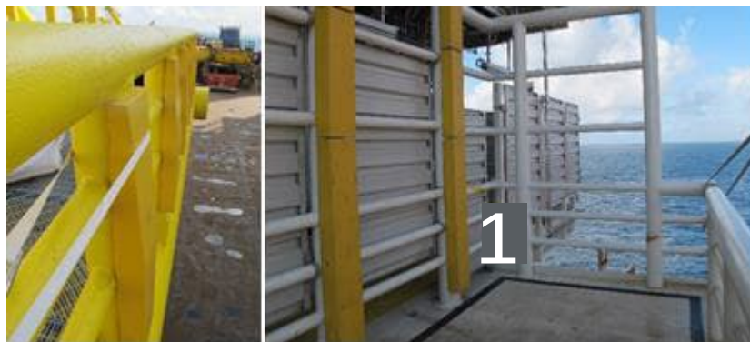
Figure 6.6 Example of bumper and guide structures
